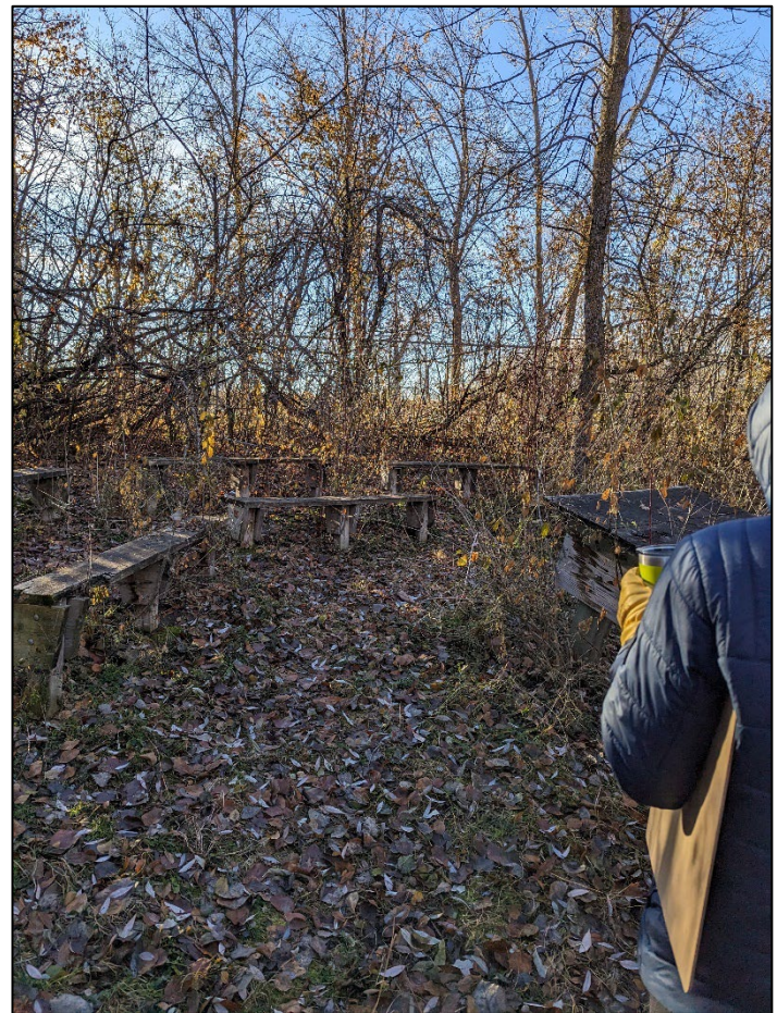
View of Outdoor Classroom Denoting The Need For Repairs And Lack of Equity Accessible Trails.
