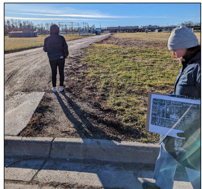
North Entrance To Highland School Off Of 3rd Ave. - View Detailing Lack of Tarred Road & No Sidewalks and Signage. Roadway Heavily Utilized By Delivery Trucks.
