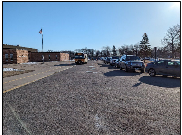
Front of Highland Elementary School Showing Bus Drop-Off Adjacent To Staff Parking.
